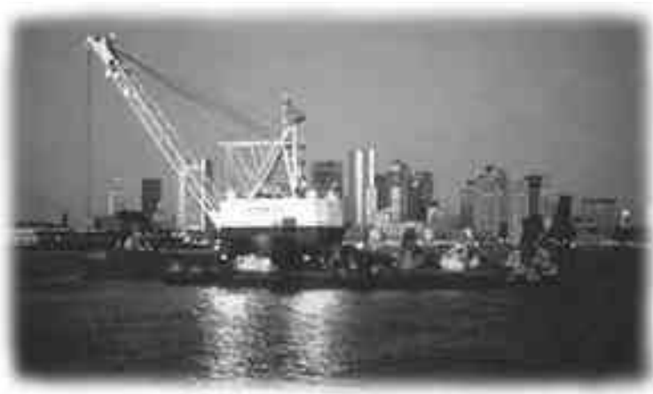
Photograph of Super Scoop provided by Massachusetts Turnpike Authority.
